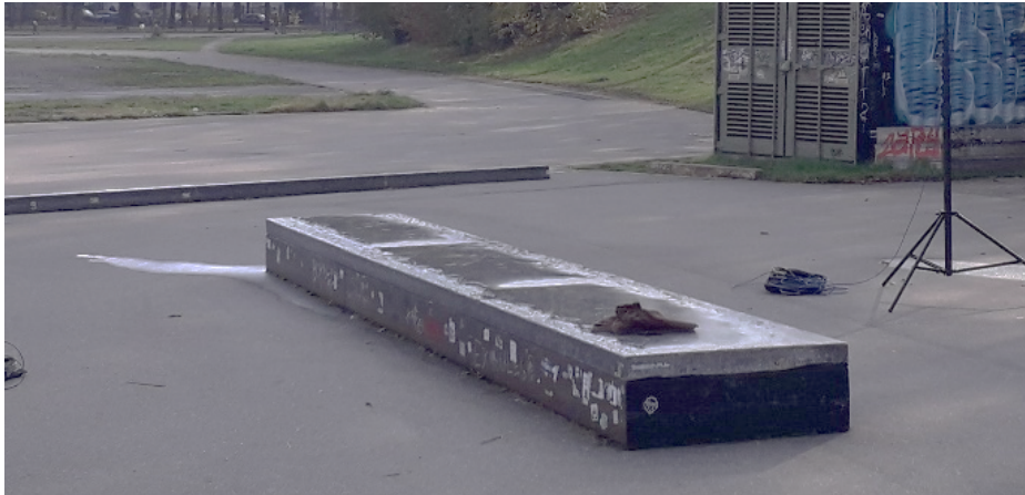
Abb. 18: Curb – Material Granit
