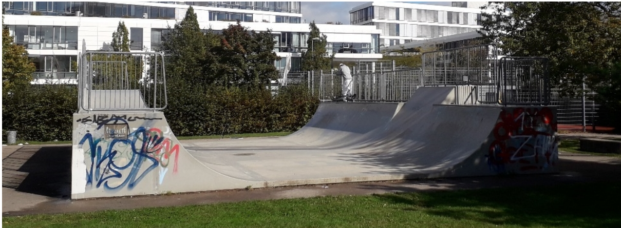
Abb. 51: Mini-Ramp – Material Beton
