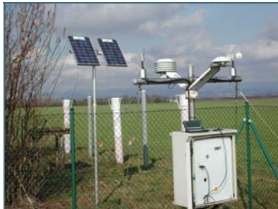
Abb. 43: Photovoltaik (Foto: LfU)
